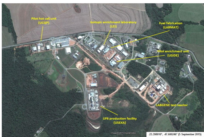
Brazilian naval nuclear facility: Aramar Experimental Center at Iperó
